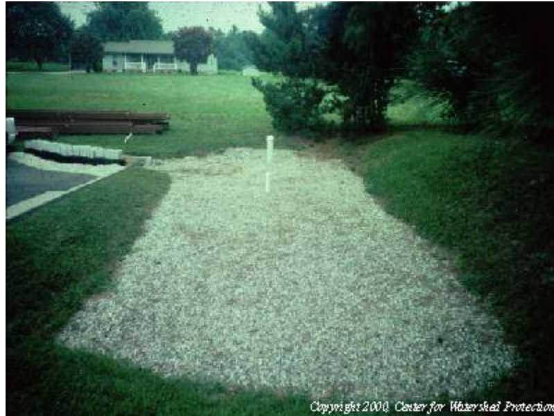
Figure PTP-05- 1 Infiltration Trench
