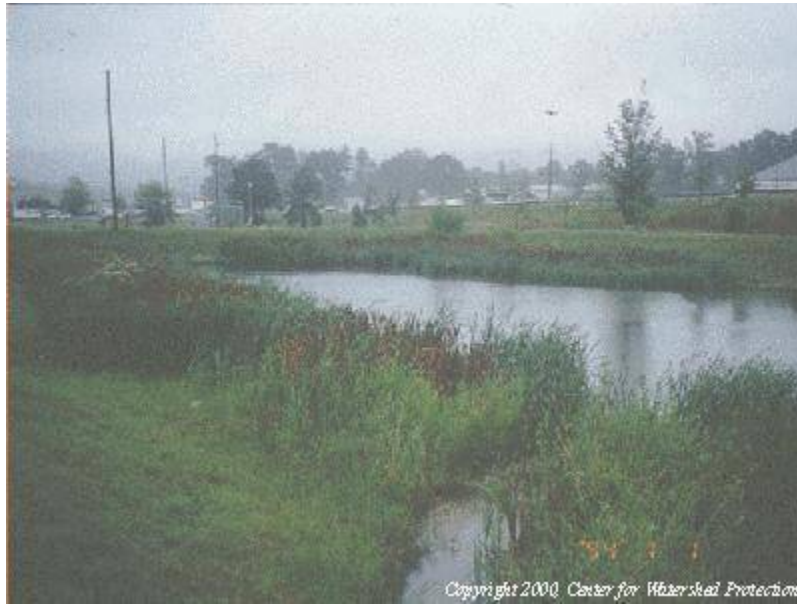
Figure PTP-03- 4 Wet Extended Detention Pond.
