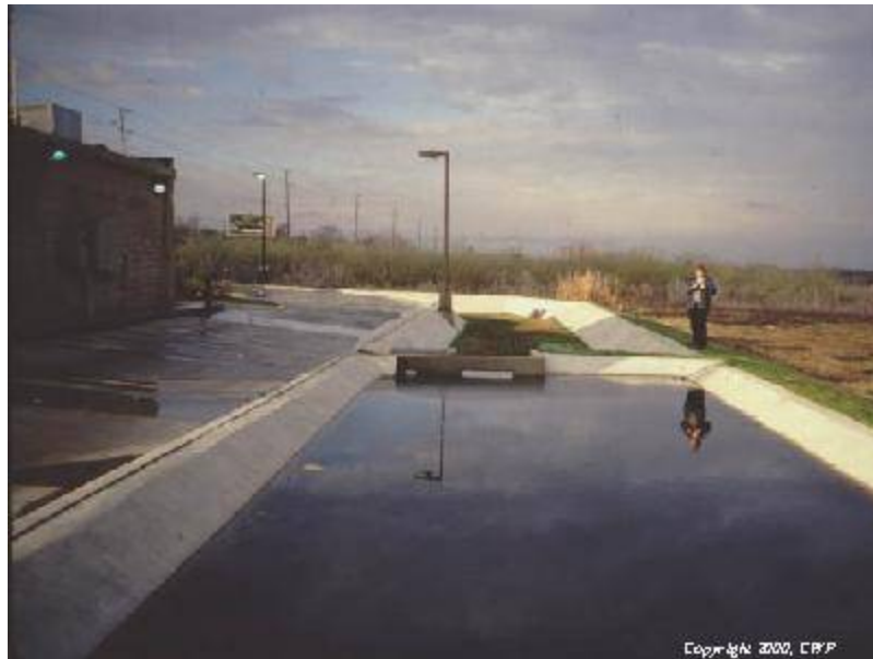
Figure PTP-01- 2 Surface Sand Filter
