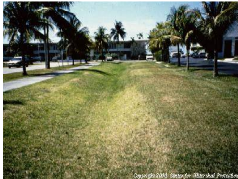
Figure PTP-02- 1 Dry Swale
