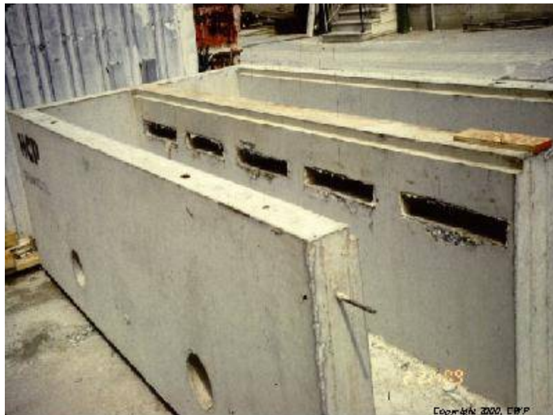
Figure PTP-01- 7 Perimeter Sand Filter
